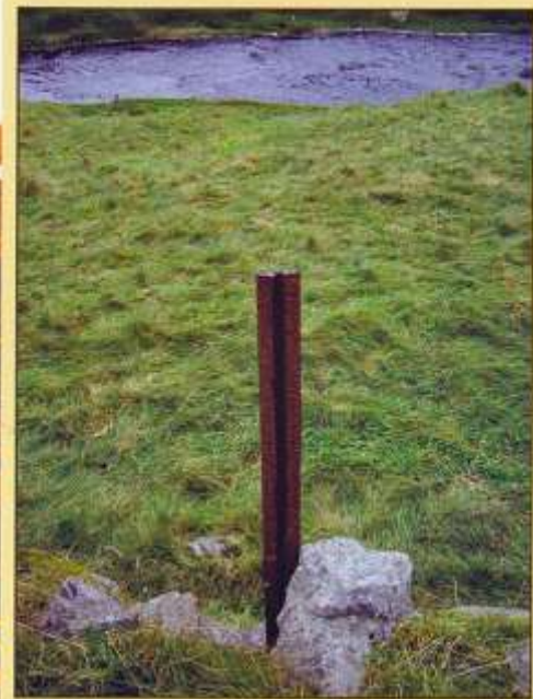
Recycled tramway line used as a fence post
